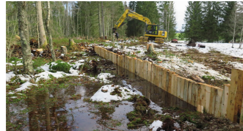
Neutralising ditches on the Cerneux-Gourinots peatland at Fournet-Blancheroche (25)
